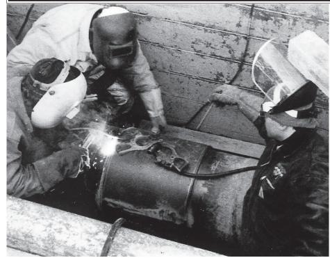
Where special precautions are needed, you can be "double-sure" of field joints by installing Dresser Style 110 and 115 reinforcing sleeves. Style 110 and 115 full-wrap sleeves are factory prepared with standard welding bevel and are machine flame cut for uniformity and ease of installation.
