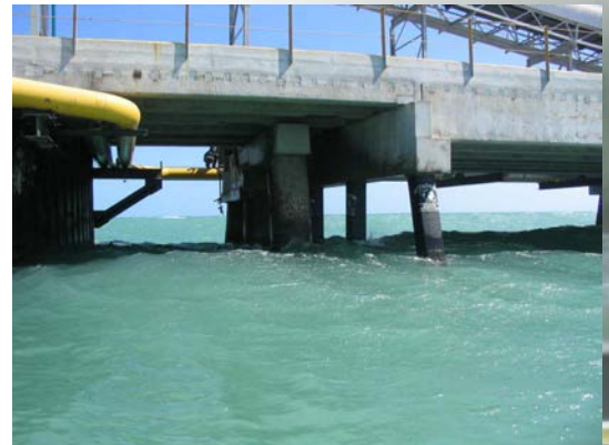
Jacket and filler blocks installed on 14" vertical and raker piles
