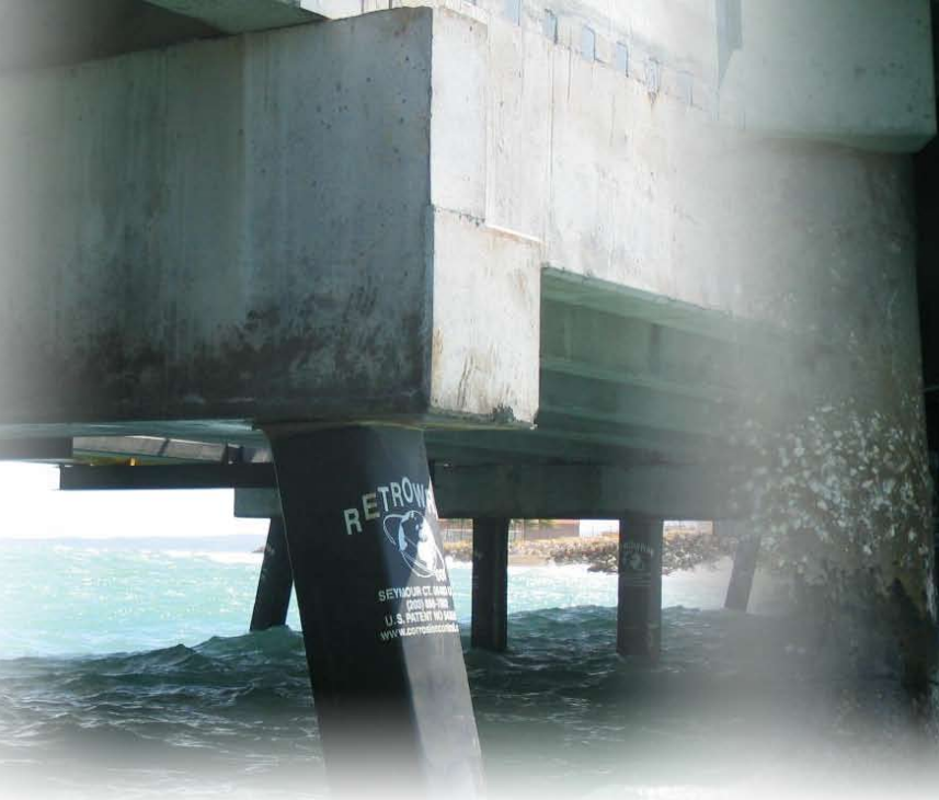
Raker pile cap termination
