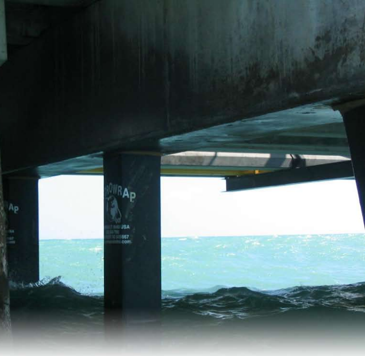
Vertical pile cap termination
