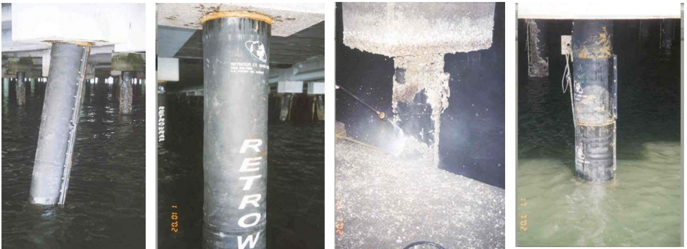
16" diameter batter pile showing outline of top seal in contact with underside of dock. Note top seal is forced against underside of pile due to hoop tension induced into fabric during installation.
