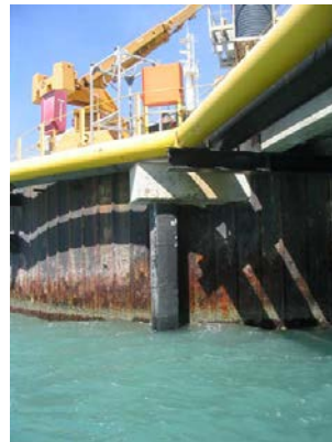
Jacket and filler blocks installed on 14" vertical and raker piles
