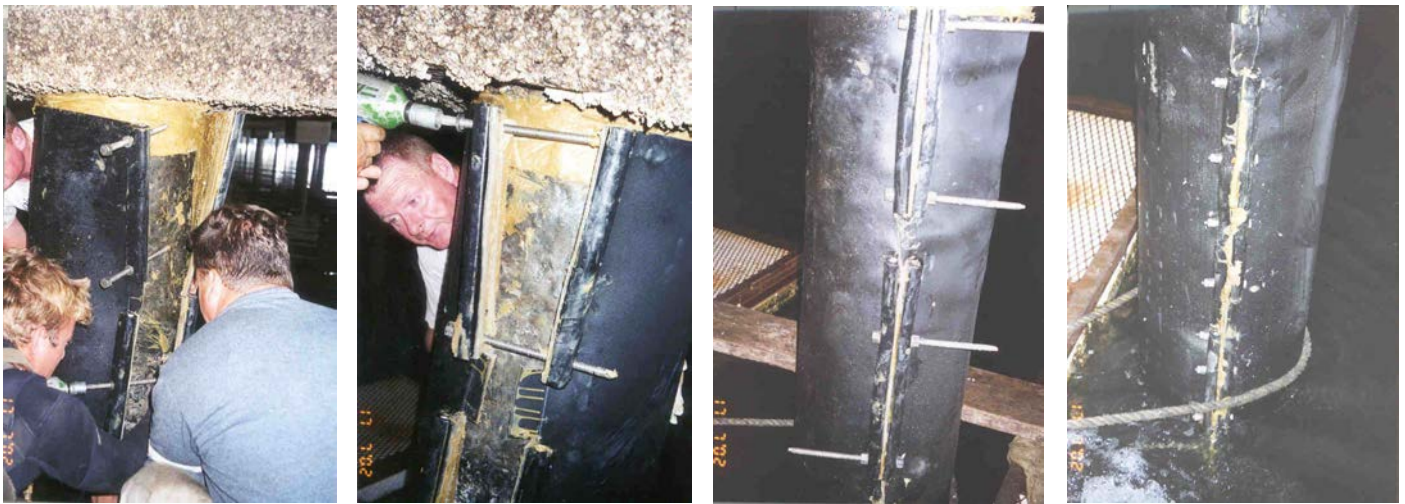
16" Retrowrap HD being secured into position.
