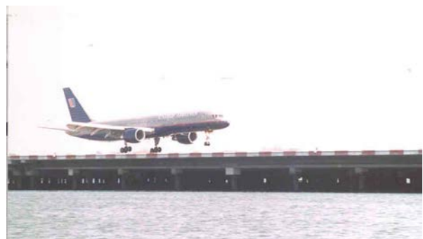
UAL757 landing on runway extension 4. 22 retrofitted piles with Retrowrap HD in foreground.
