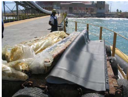
Full length one piece outer jacket with lag fasteners pre installed. Note Indent tag attached to jacket to ensure correct installation
